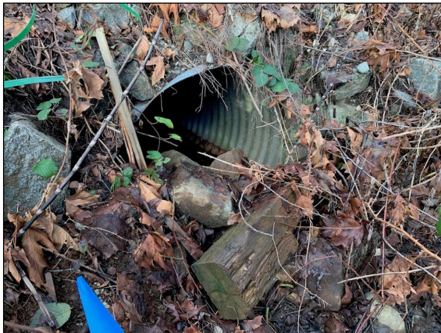
Photograph 6: Northward view of the inlet of Culvert 1. Culvert 1 is a 1200 mm corrugated steel pipe. Photograph taken January 19, 2021.
