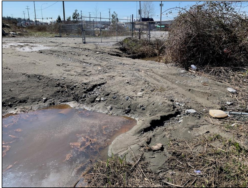
Photograph 27: Southwestern view of the new vehicle crossing located near the downstream end of the Wetland Channel showing the inlet of Culvert 2. Photograph taken April 8, 2021. Note Culvert 2 has since been removed by neighbouring property owner.
