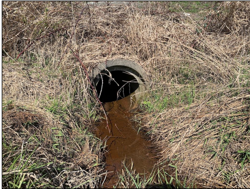
Photograph 43: Northward view of the inlet of Culvert 8 at Old Yale Road which conveys the flow from the Off-Site Wetland Channel. Culvert 8 is a 600 mm diameter concrete pipe. Photograph taken April 8, 2021.
