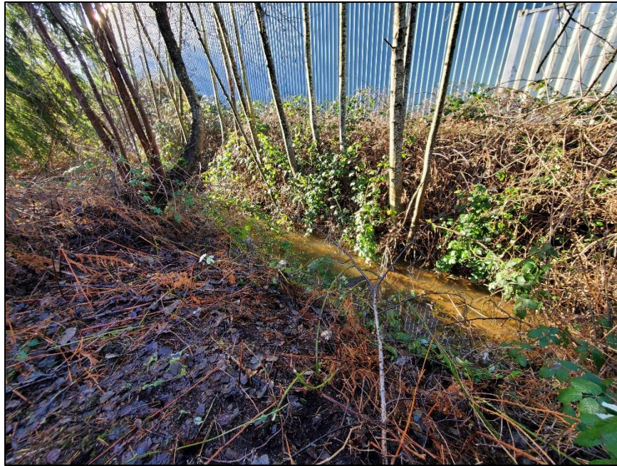
Photograph 11. Westward view of the conditions at the northern portion of South Stream 2. Photograph taken January 19, 2021.
