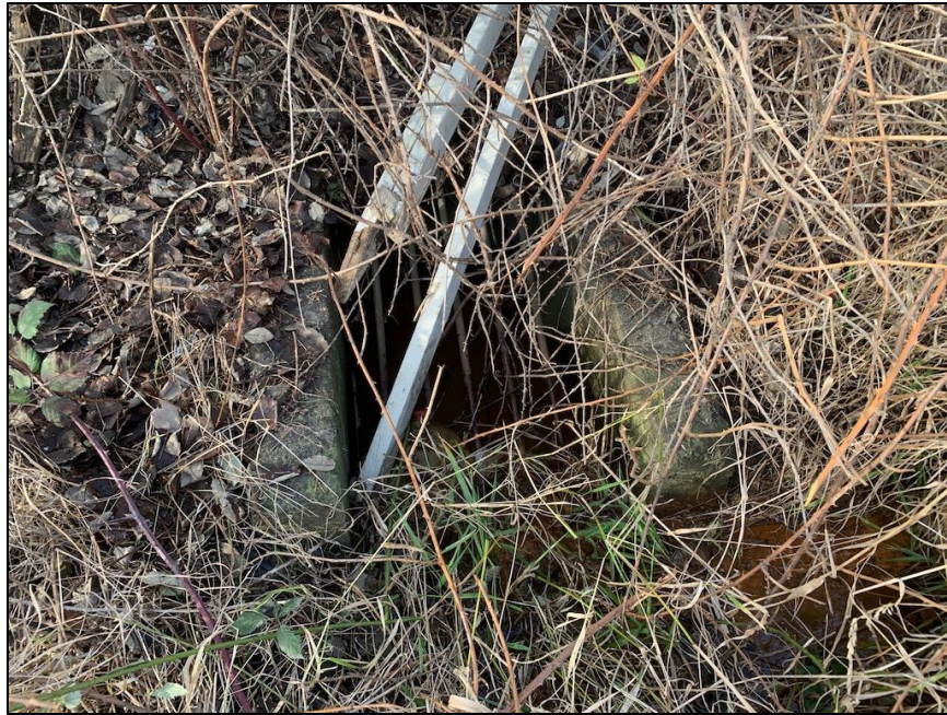
Photograph 35: Westward view of the inlet of Culvert 4 located at the northern end of Ditch 1. Culvert 4 conveys drainage west under Scott Road. Photograph taken January 19, 2021.
