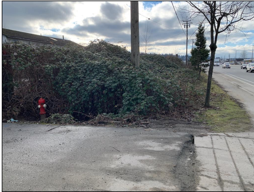
Photograph 41: Southward view of the downstream end of Ditch 3 at Culvert 7 under the driveway for the property to the north of the Site. Photograph taken January 19, 2021.
