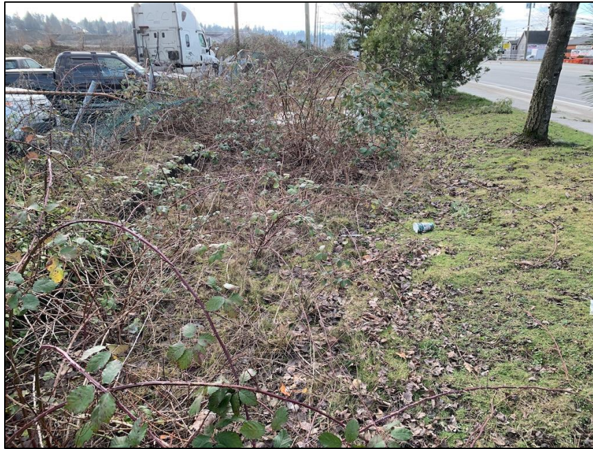
Photograph 37: Southward view of the slight depression along the boulevard west of the central property at 10582 Scott Road. Photograph taken January 19, 2021.
