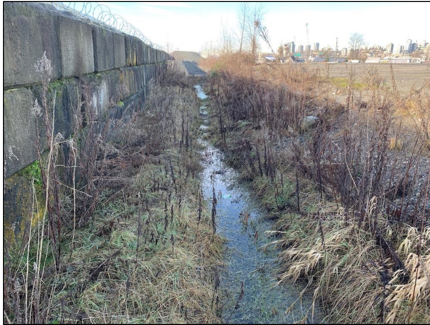
Photograph 33: Westward view of the western portion of the South Ditch. Photograph taken January 19, 2021.
