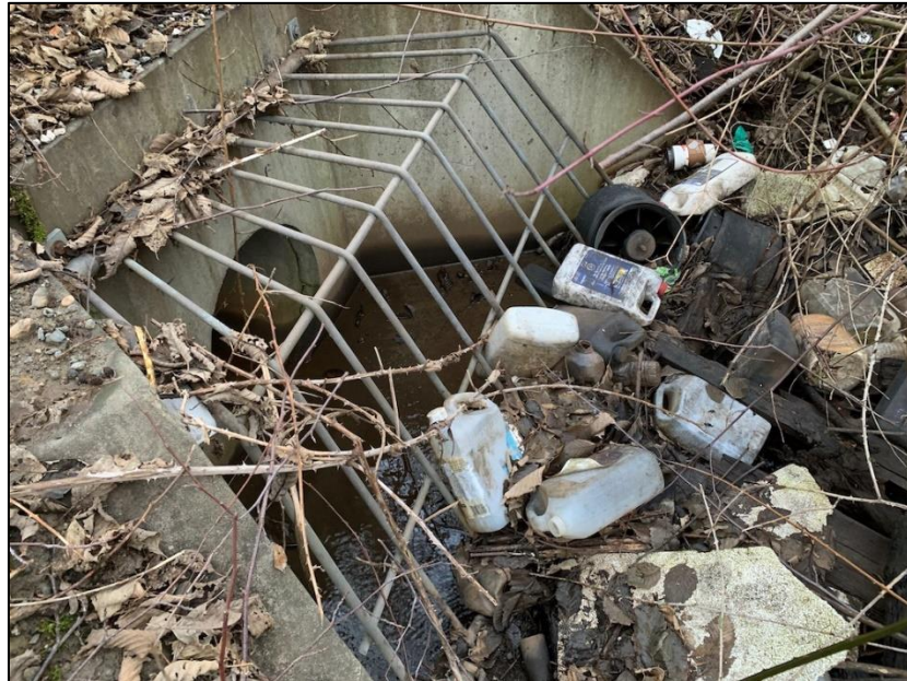
Photograph 46: Inlet of Culvert 10 at the outlet of the Constructed Habitat Pond at the north end of the pond. Culvert 10 is a 600 mm diameter concrete pipe. Photograph taken January 19, 2021.
