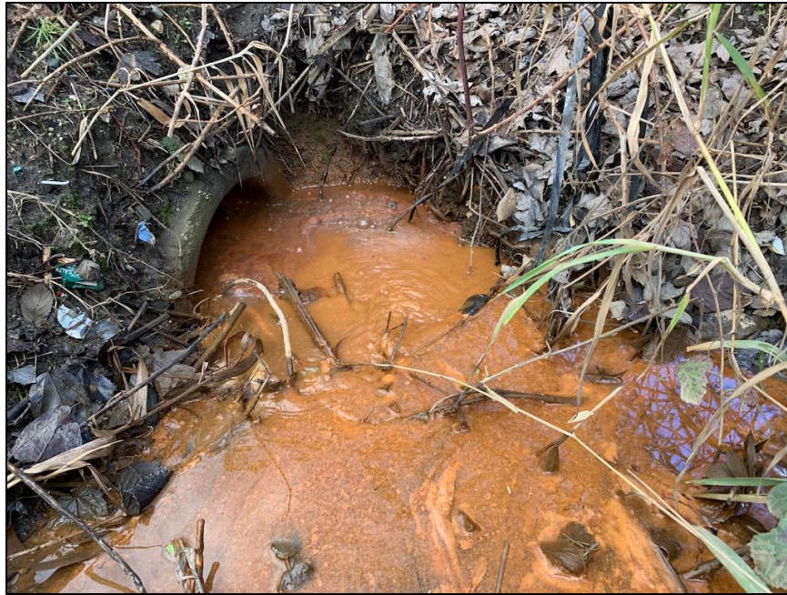
Photograph 31: Inlet of Culvert 3 at the downstream end of the Wetland Channel. Culvert 3 drains into the northern end of Ditch 1. Photograph taken January 19, 2021.
