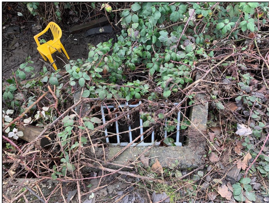
Photograph 42: Inlet of Culvert 7 at the north (downstream) end of Ditch 3 at the driveway for the property to the north of the Site. Photograph taken January 19, 2021.
