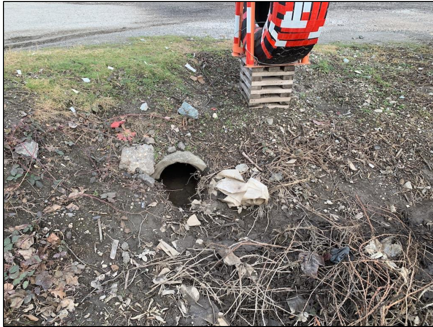
Photograph 39: Northward view of the inlet of the 300 mm diameter concrete pipe (Culvert 6) at the downstream (north) end of Ditch 2. Photograph taken January 19, 2021.
