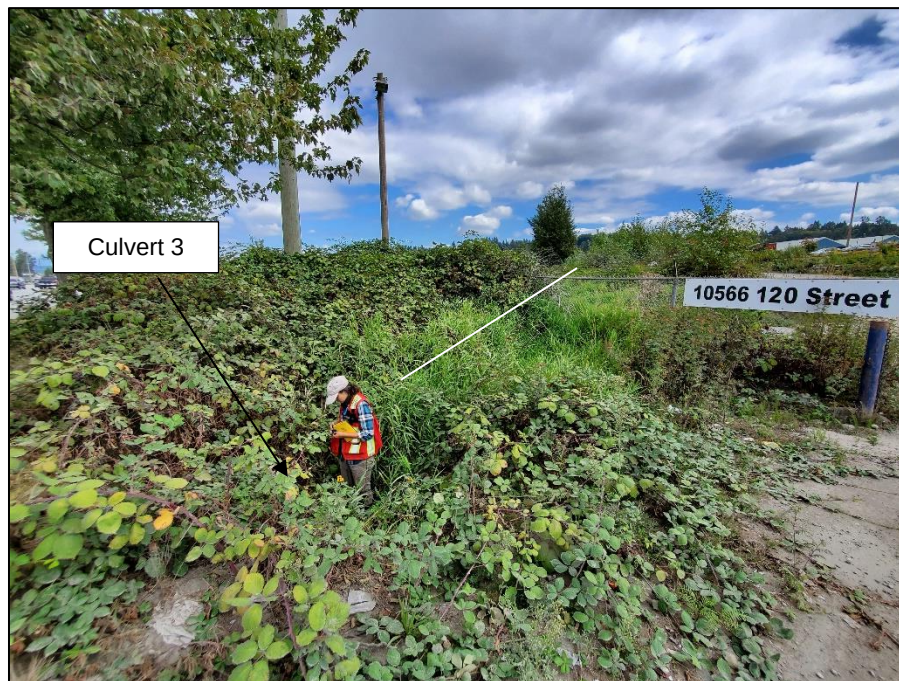
Photograph 30: Eastward view of the Wetland Channel at the inlet of Culvert 3. The white line shows the alignment of the Wetland Channel. Photograph taken September 1, 2020.
