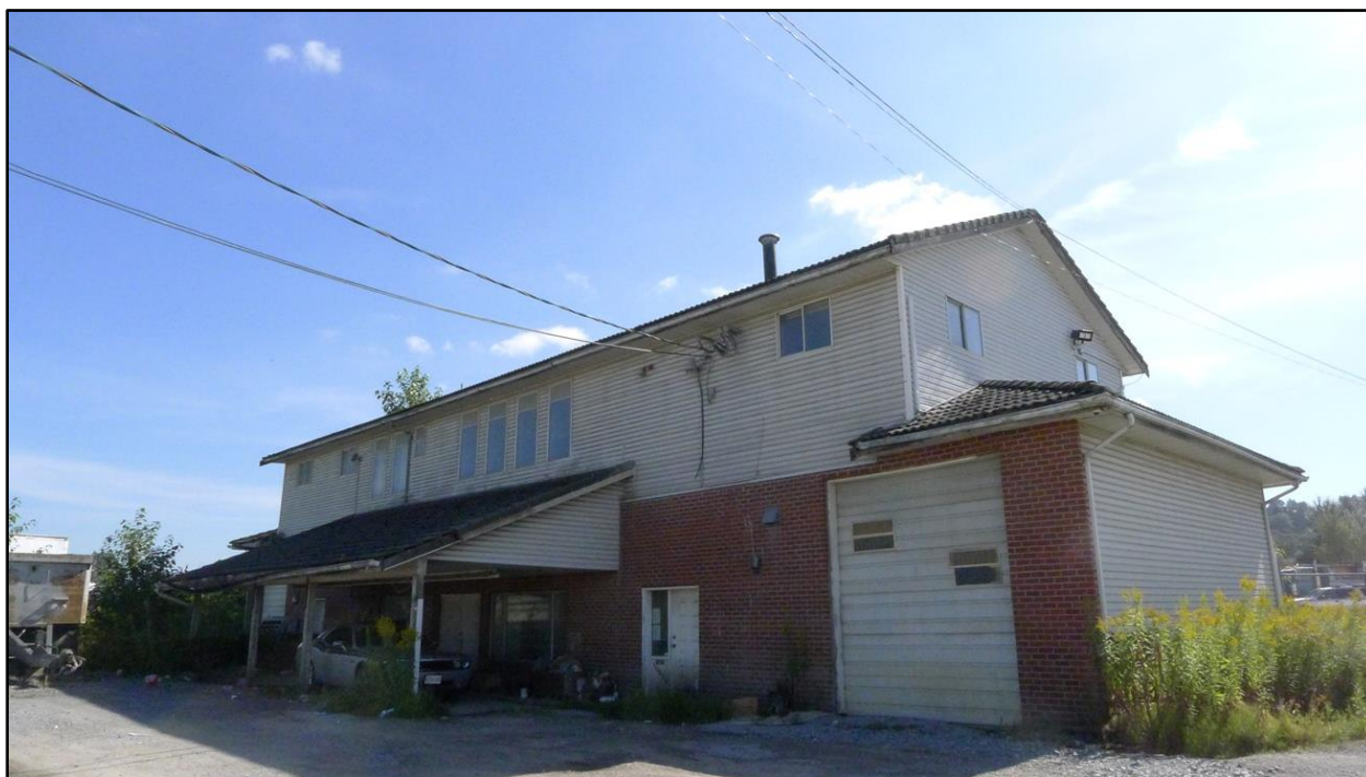
Photograph 5: Residence on the northwest portion of 10626 Scott Road looking northeast
