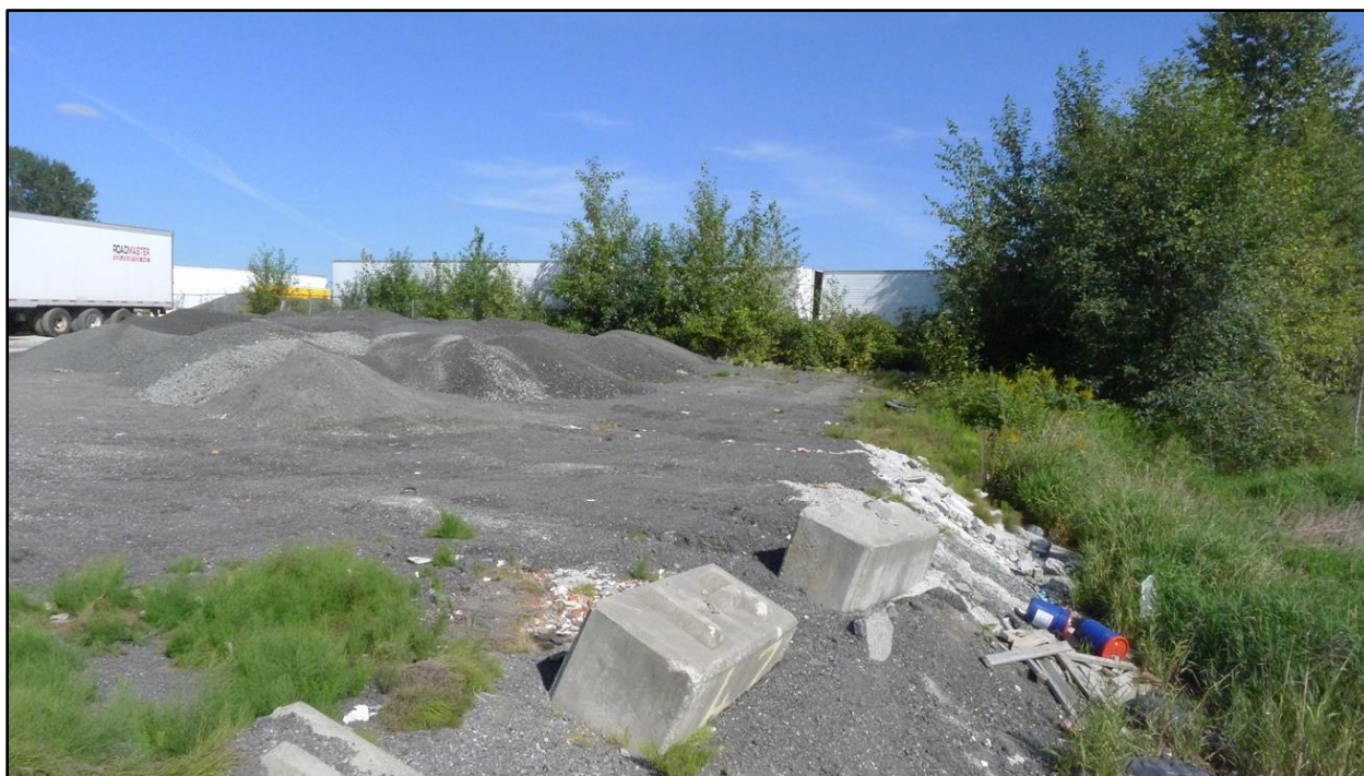
Photograph 7: Fill material and lubricant container disposal at the centre of 10620/10626 Scott Road looking north
